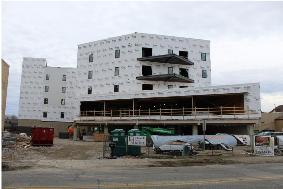
NOVA Towers, 200 S. 4 th Street, Lafayette, IN
